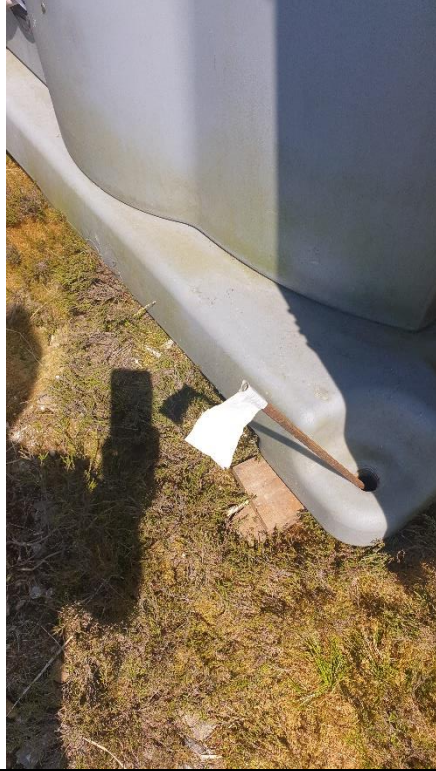
South-east ground anchor
