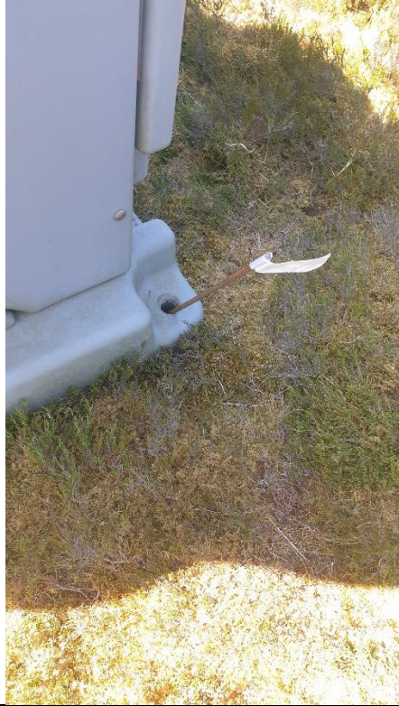
North-east ground anchor
