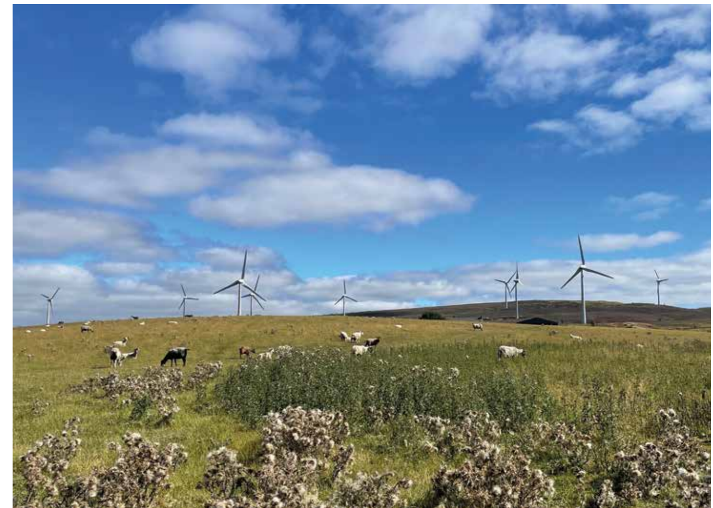
Berry Burn Wind Farm, Forres in Moray. 29 turbines, 100m tip height
