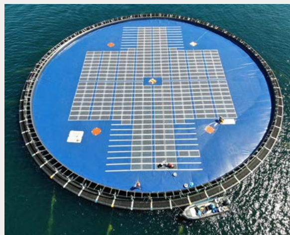
Floating solar system, Statkraft plant in Albania. R&D project. Concept developed by Norwegian company Ocean Sun. This solution requires little material per kilowatt. Each unit basically consists of only a membrane, plastic floating rings and anchoring equipment, and the solar panels.
