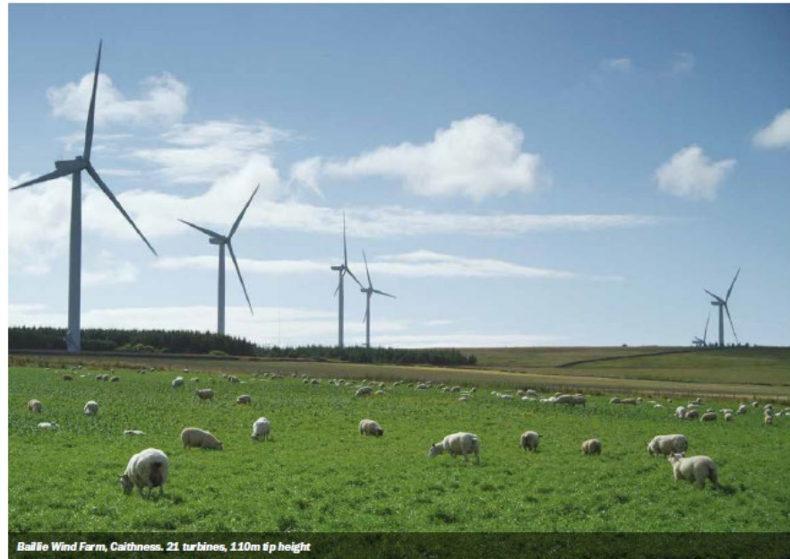
Ballis Wind Farm, Caithness. 21 turbines, 110m tip height
