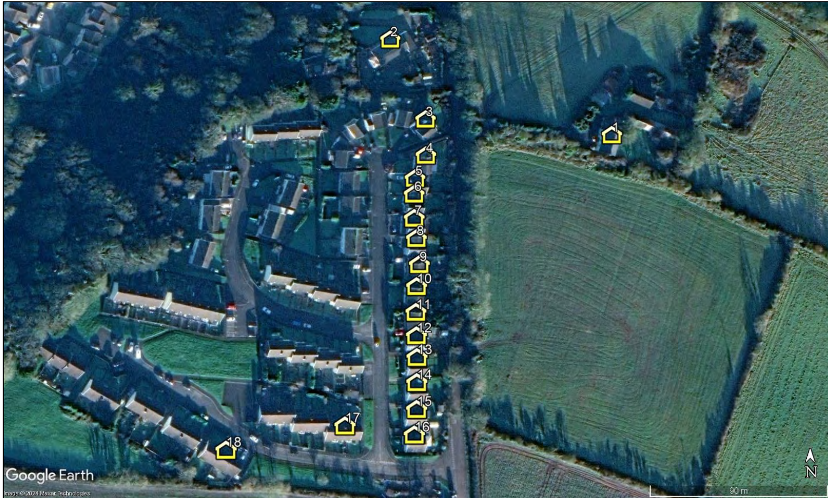
Figure 5 Assessed dwelling receptors 1-18 - aerial image
