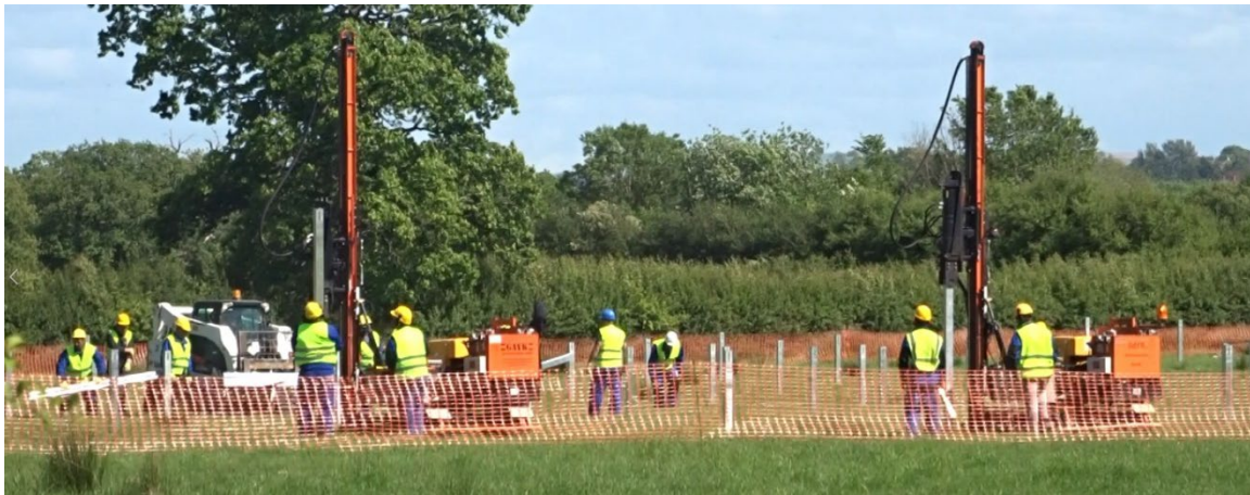
Photograph 11: Example of piles Being Delivered and Installed
