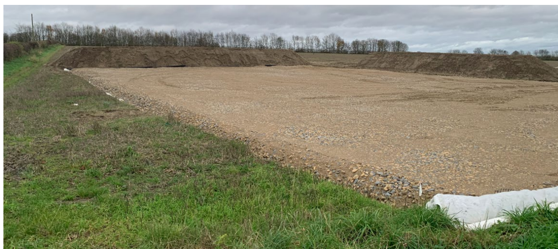
Photograph 23: Newly-laid Construction Compound (Elsham-Lincoln Pipeline)
