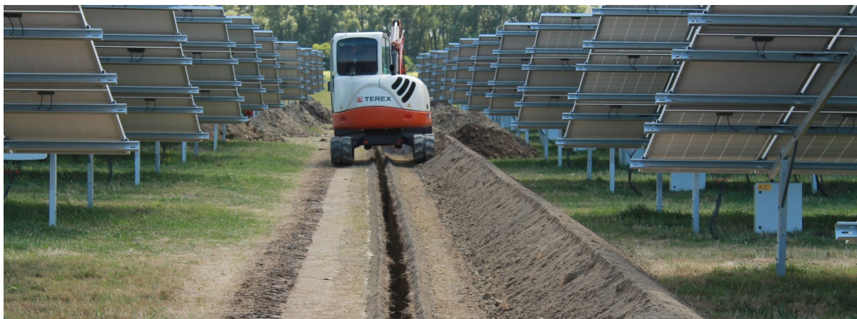
Photograph 20: Cable Trenching, Central Row
