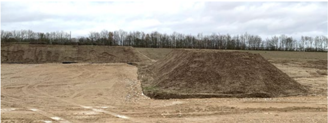
Photograph 25: Topsoil Storage Bund
