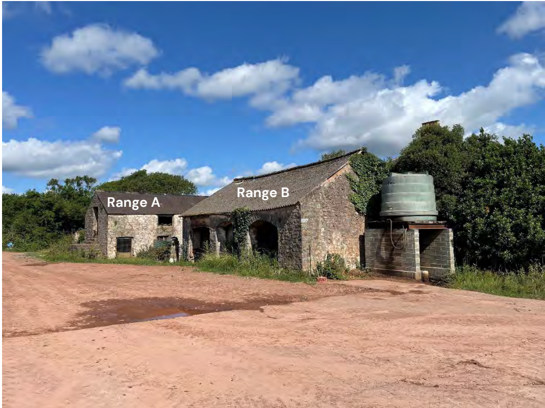
Plate 1: Historic outbuildings to the rear (south) of Alleston Farmhouse, looking north-west from where the farm access track enters the farmyard
