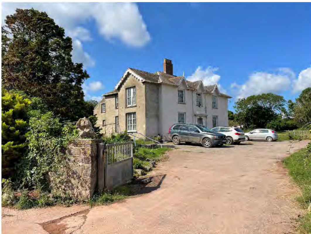
Plate 10: Close-ranging view of Alleston Farmhouse (east- and north-facing elevations) from its driveway
