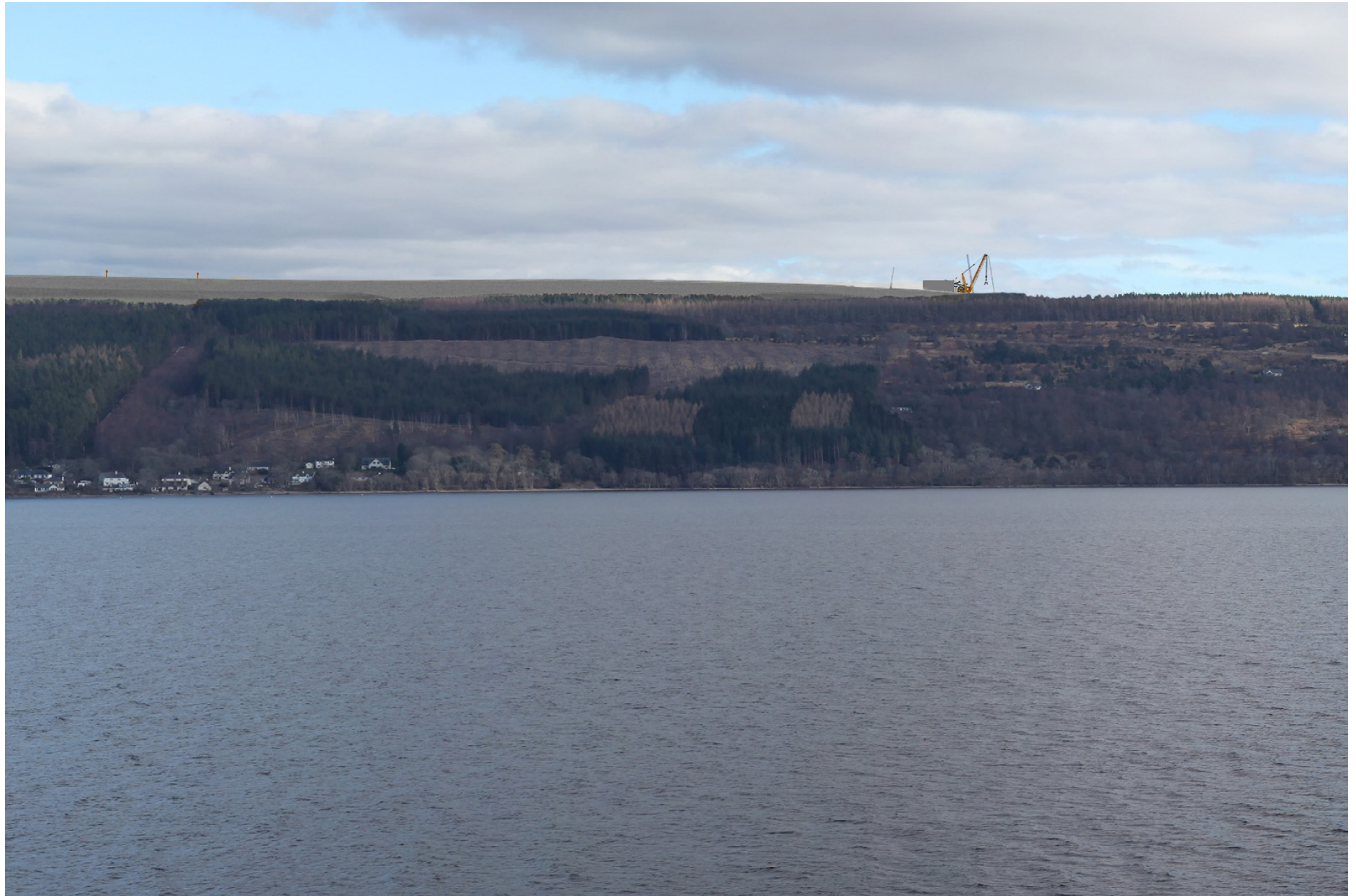
Viewpoint 10 - Layby on A82 Photomontage during construction, Year 5 Headpond Construction, 75mm Focal Length
