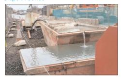
Where there are constraints on space that prohibit the use of construction SuDS (i.e. settlement lagoons as described above) an alternative option might be to drain runoff through a series of skips filled with clean aggregate or straw bales to encourage filtration and settlement of suspended fine particulates.
