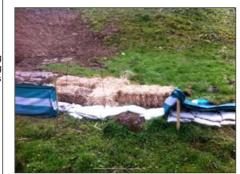
Like fabric silt fences and sand bags, straw bales are a multipurpose way to manage construction site runoff to prevent untreated ingress to water bodies and to support the filtration of fine particulates from runoff.
