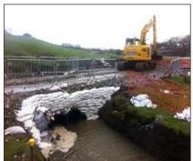
Sand bags provide a flexible way to prevent sediment-laden runoff entering a watercourse by creating temporary dams and barriers to runoff. This is most effective on the face of temporary watercourses crossings and short length land depressions where there are preferential flow pathways.
