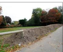
These are temporary barriers to conveyance of construction runoff and can be used to create temporary storage lagoons or barriers between construction works and water bodies. Care needed as earth bunds may themselves be a source of fine sediment, although this can be minimised by covering with a suitable geotextile or seeding if they are to be in place for a longer period of time and not part of topsoil storage.
