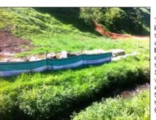
These are geotextiles installed in the path of sheet flow runoff to filter out sediment. They are often installed around water bodies, below the toe of a cleared slope or around temporary earth stockpiles. Silt fences detain sediment-laden water and promote settlement and may remove 80-90% sand, 50-80% silty loam, and up to 20% silt-clay loam in runoff (CIRIA 648, 2006).
