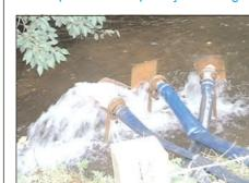
If the rate and energy of temporary discharges are not controlled there is a risk of eroding the bed and banks of the receiving water body. The use of baffle pads on the outfall is one way in which the energy of the outfall can be dispersed to avoid bank and bed erosion.
