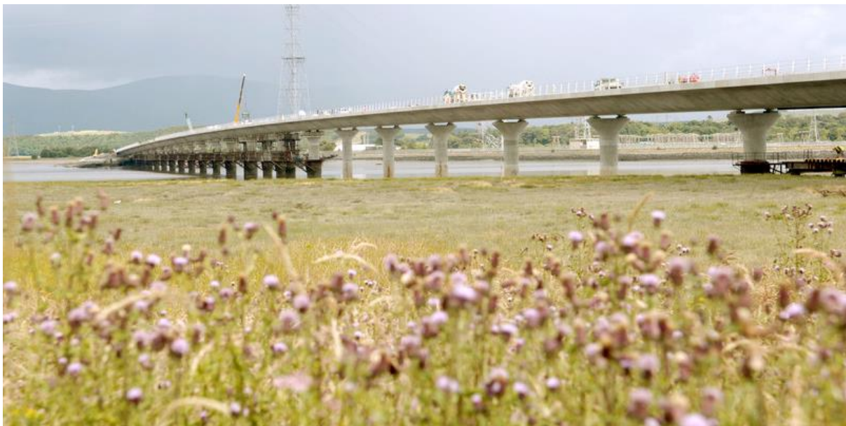
Bridge maintenance (courtesy of SEPA)
