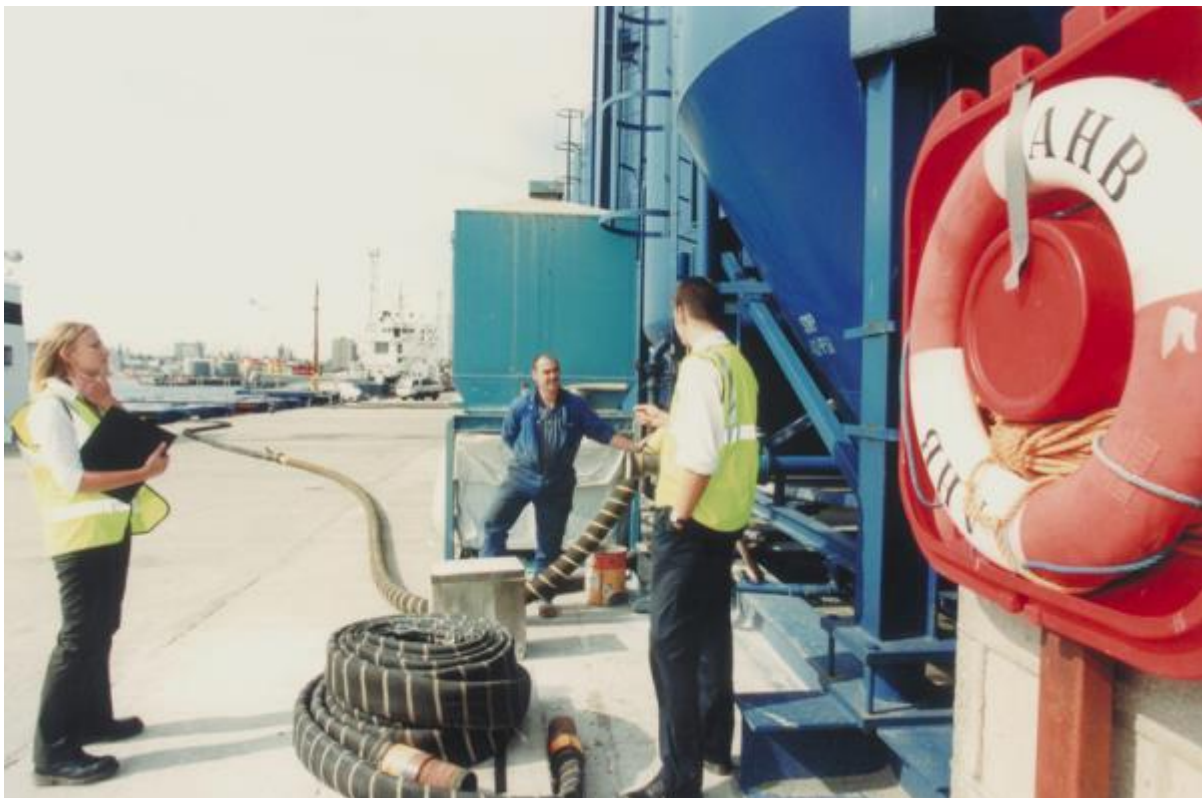
Cement silo inspection (courtesy of SEPA)
