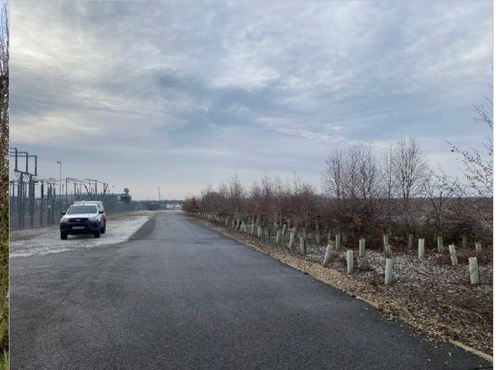
IMAGE 3: Looking south along the west side of the substation with an area of new tree planting to the right of frame.
