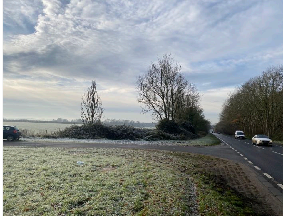
IMAGE 1: Looking south across the existing substation access onto the A47
